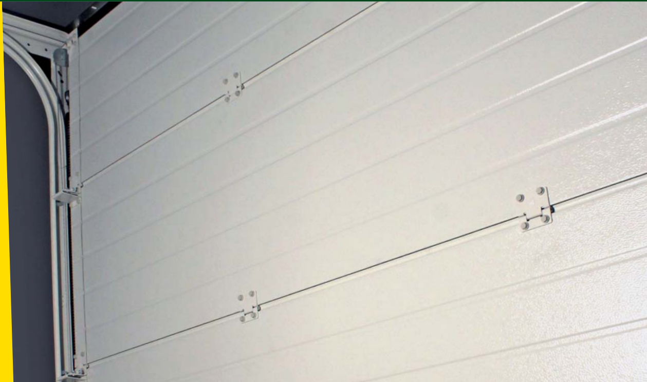
Vertical Traction Springs placed between rails and jambs.
