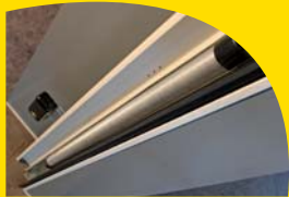
Vertical Traction Springs placed between rails and jambs.
